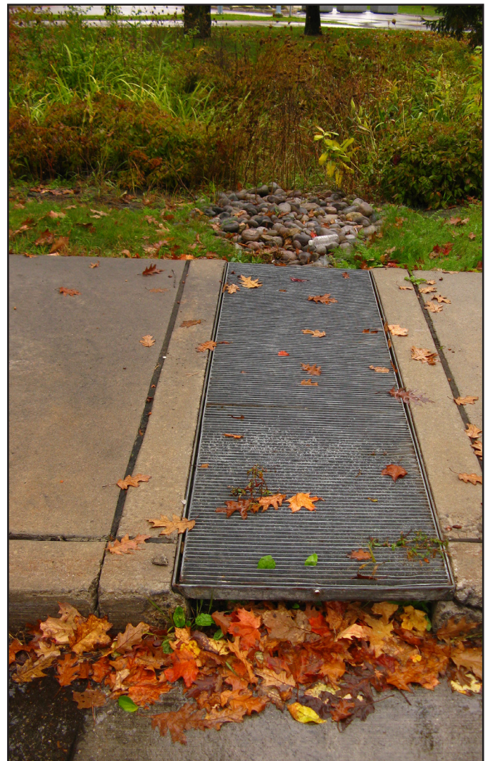
Figure 5. Leaves clogging inlet to bioretention
