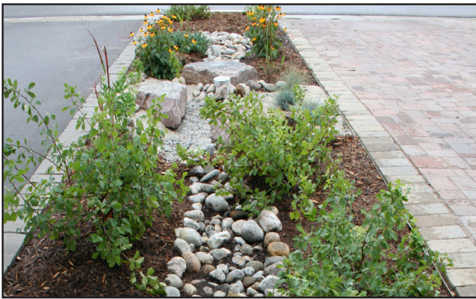
Figure 1. Bioretention in residential area
